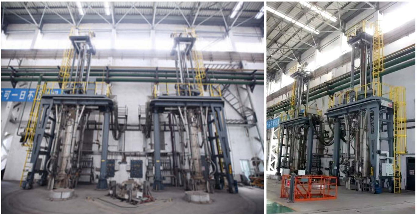
18 tons German ALD gas protection ingot electroslag furnace
